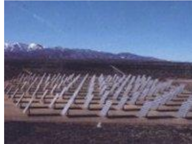
1MW Arco Solar – Solar Park, Hesperia, California
