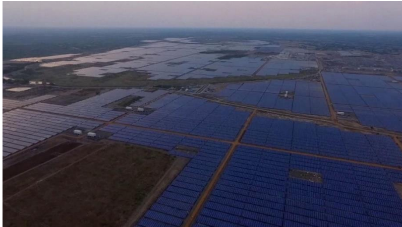
Adani's 648MW Solar Farm in Kamuthi, Tamil Nadu
